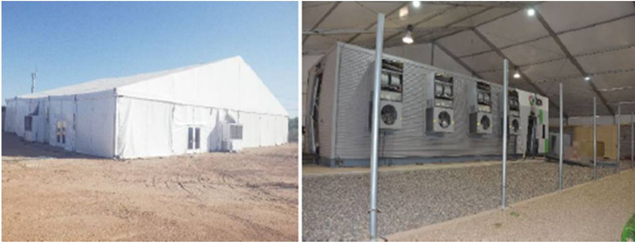
Figure 10 Climate controlled tent structure erected by APS to preserve the BESS site during the investigation (image credit: APS)
